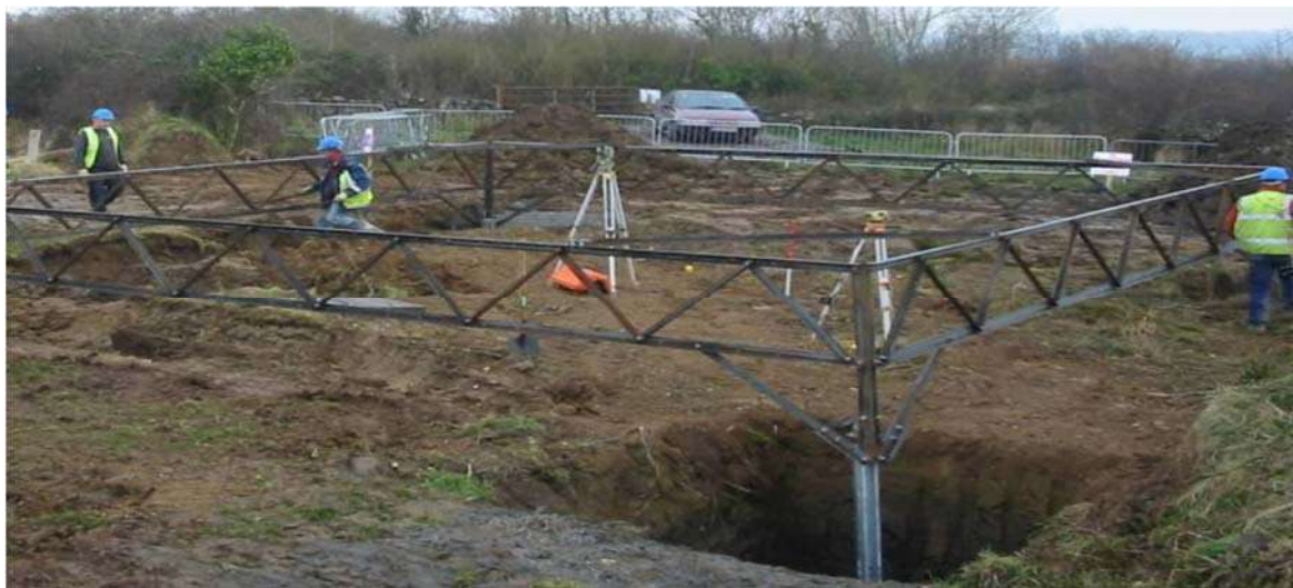
Figure 2.3 Photograph setting template being prepared for final concreting
