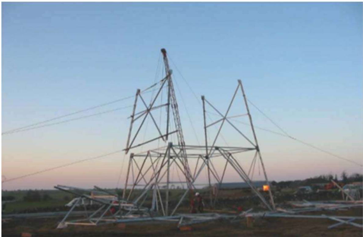
Figure 2.4 Model visual: Derrick pole at tower base
